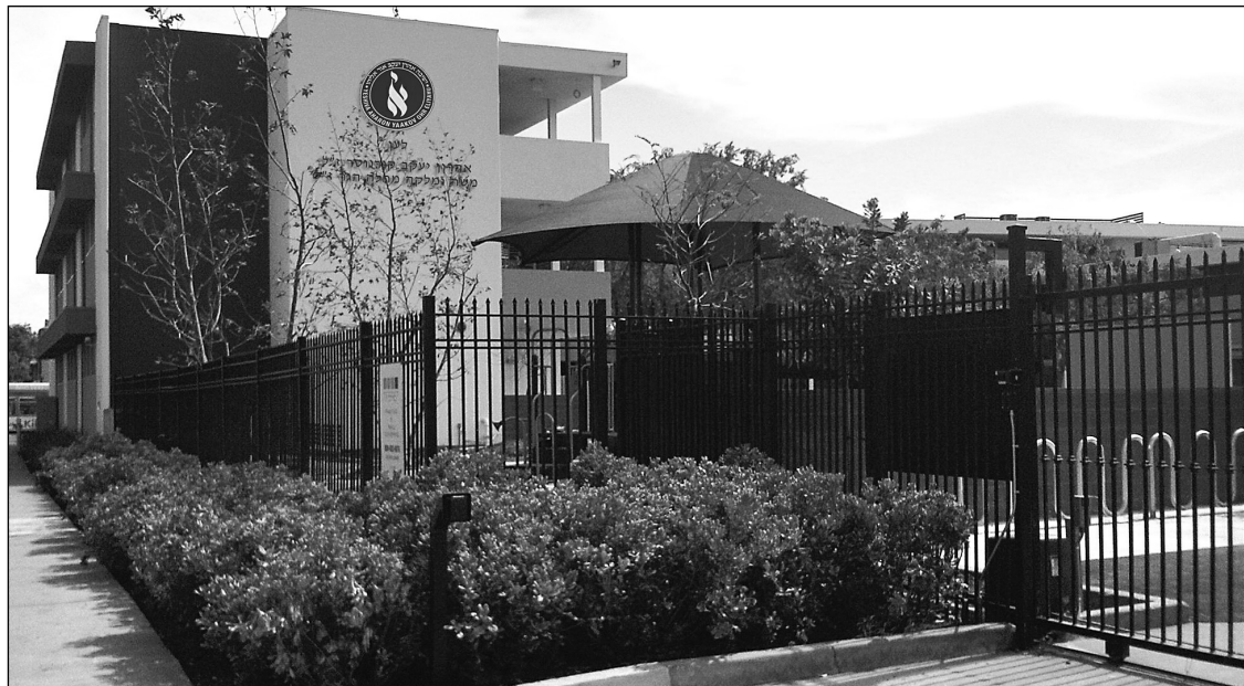
The yeshivah building
